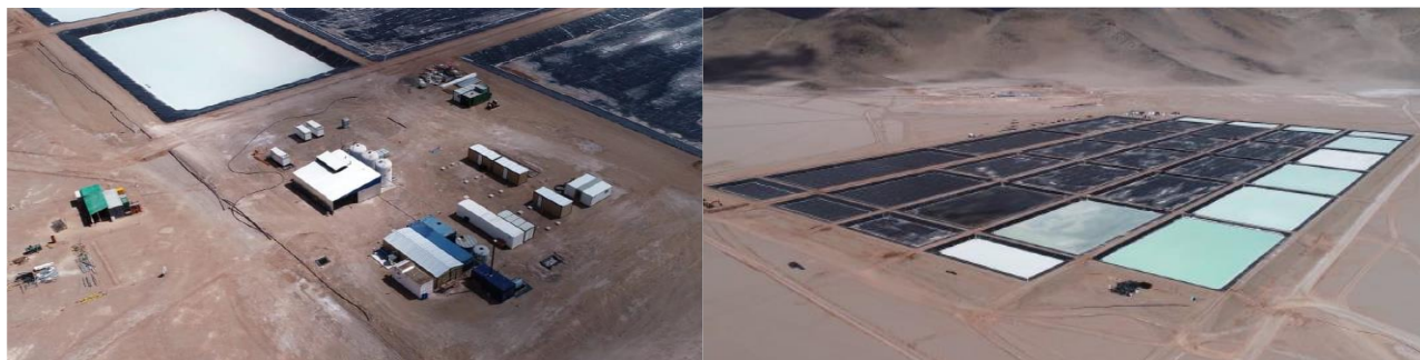
Figure 1: Completion of pilot plant construction (left) and over 30% of pilot pond were filled with brine (right) at the end of the quarter
